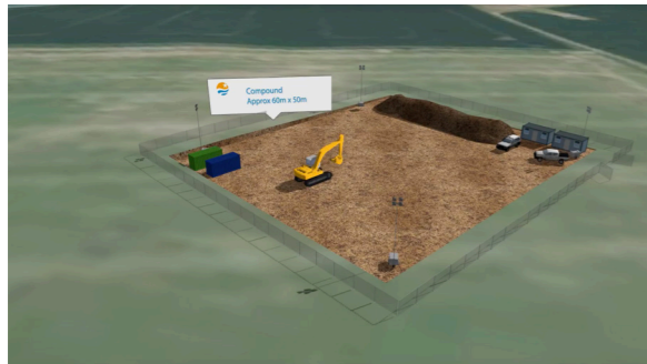
1. Site establishment including topsoil strip and store
