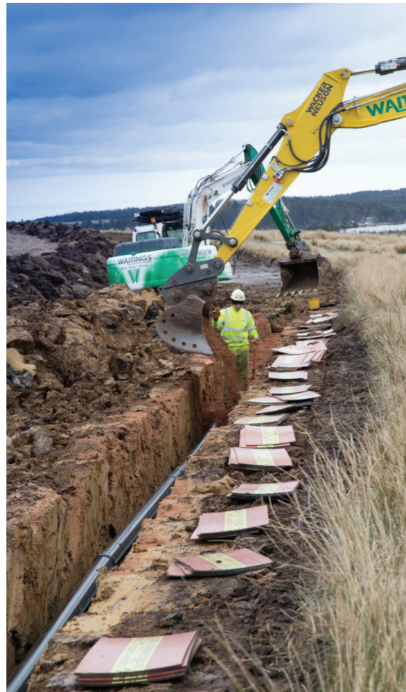
3. Ducts Covered and Protective Marker Tiles Laid
