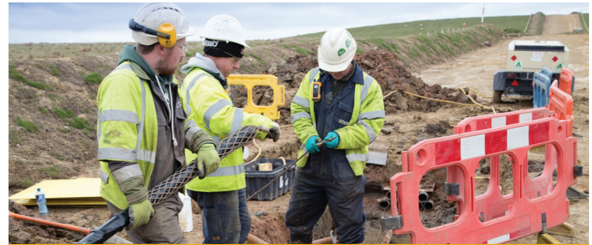
Cable pulling preparation
