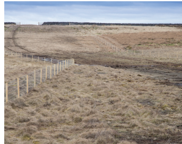
5. Reinstate Topsoil
