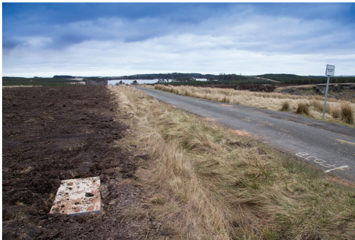
Cable easement post reinstatement, with link box at field boundary
