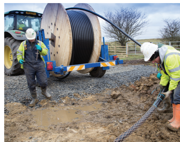
7. Pull cables into ducts
