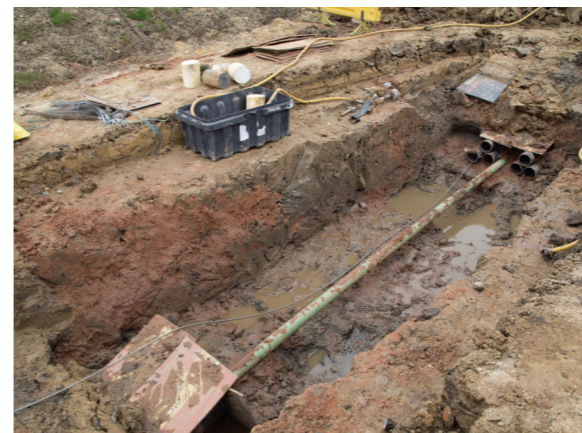
6. Excavate Joint Pit and Conduct Cable Pull (Post Duct Installation and Reinstatement)
