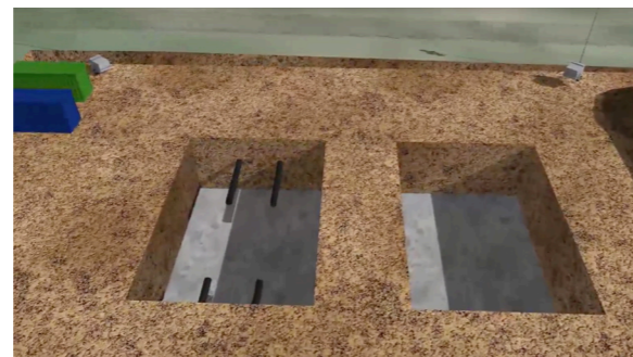
5. Cable pulled through ducting and jointed
